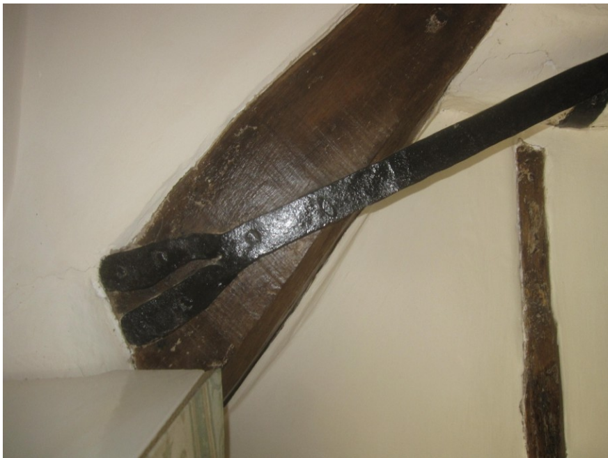
Detail of iron reinforcing strap to truss T1
