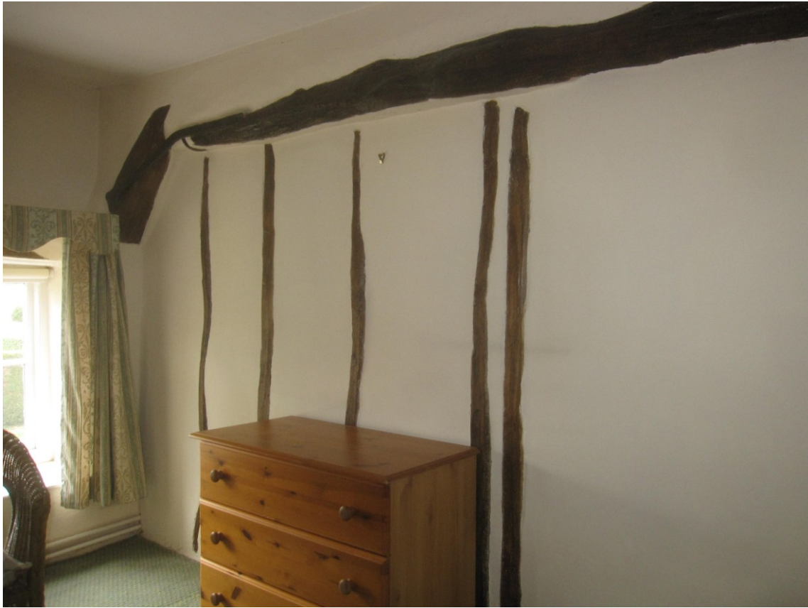
Truss T1 with stud partition, north face
